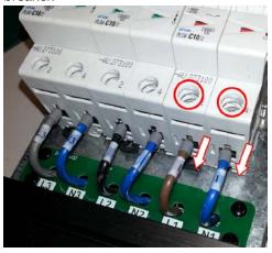
2. Cut the crimped ferrule off each wire.
