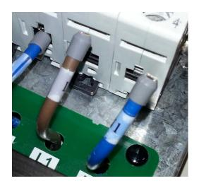
3. Remove the plastic remaining from the ferrules and strip the wires (approximately 8-10 mm).
