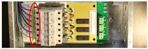
7. Recheck all terminal screws and tighten.
